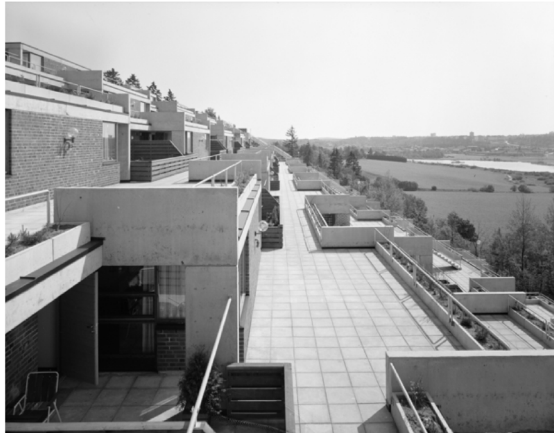
1980 - Oppsal terrace houses.
